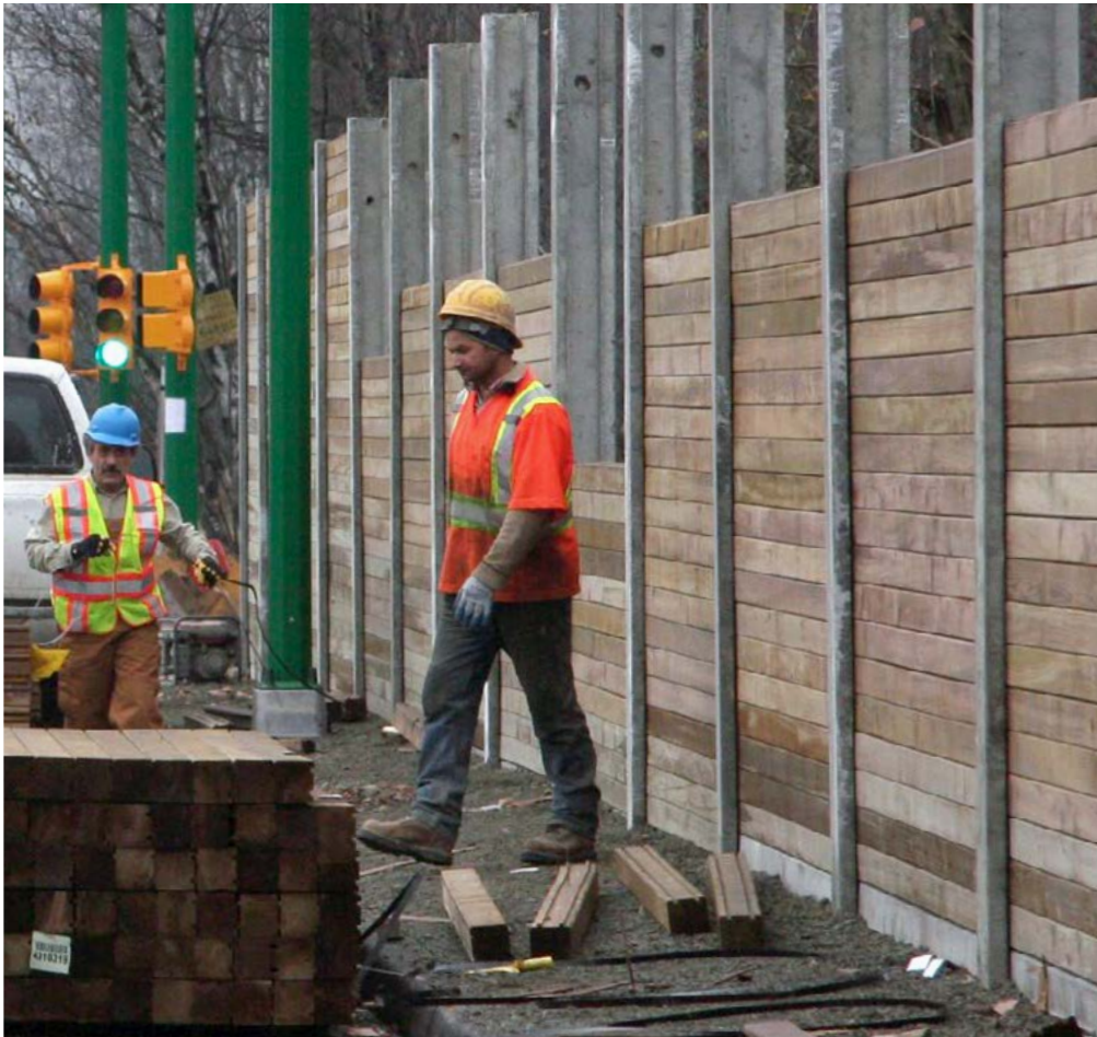
A 3-metre-high Pacific HemFir SoundShield installation in progress. Image courtesy of FPIInnovations
